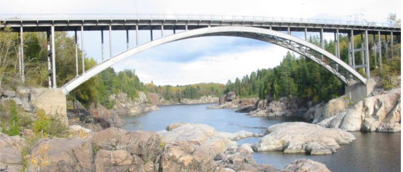
The Arvida Bridge, in Quebec, Canada was the first transport bridge in the world constructed in Aluminium in 1950. This bridge is still in use today.
